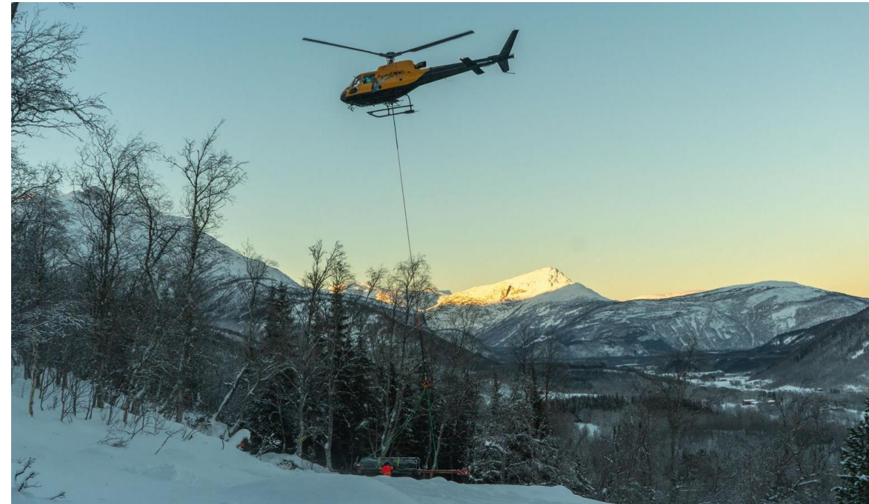
Photo: Drill rig assembly at the Lille-Leiden Project, Norway
